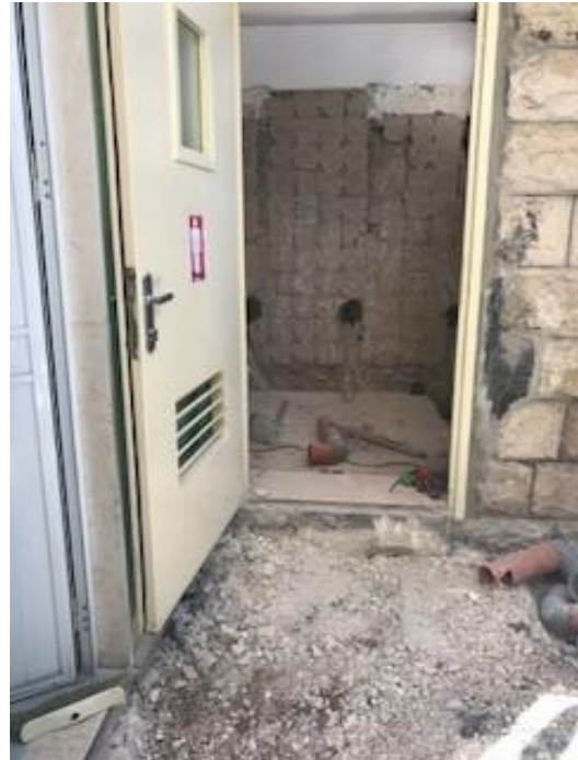
Rawdat Al Zohour-East Jerusalem - During Interior structure improvements implemented
